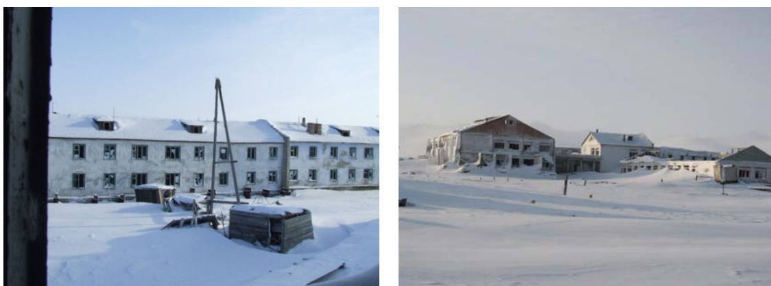
Photograph 2. Abandoned settlement Polyarny
