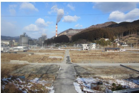
Photo 6: Oikata Area and the Factory of Taiheiyo Cement Corporation in Akasaki District Note: Photo by author, Jan. 29th, 2013.
