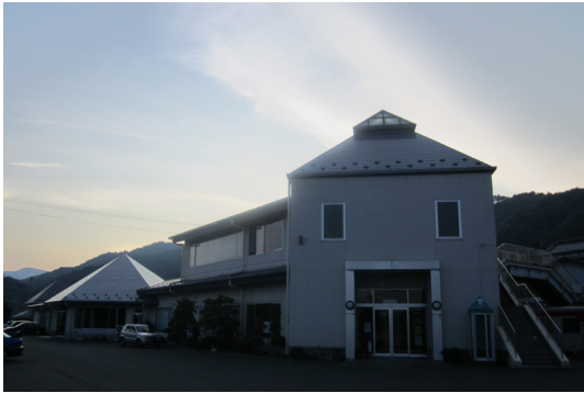
Photo 3: Yoshihama District Community Center. Note: Photo by author, Aug. 23rd, 2012.
