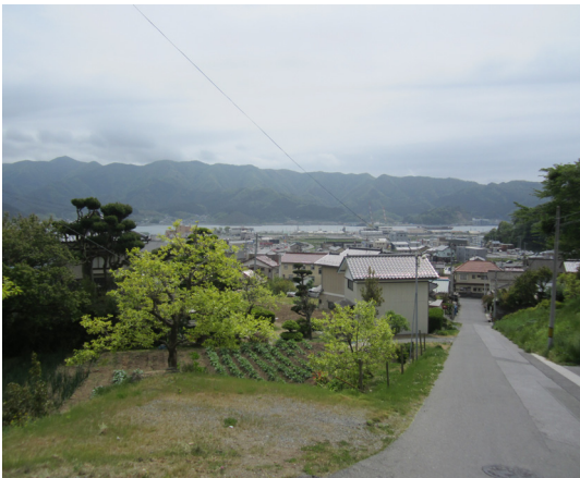
Photo 12: Slope from Center Core to Ofunato District Community Center Note: Photo by author, May 27th, 2013. Under the slope, houses and buildings were totally flooded. On the middle of the slope almost half-collapsed or partially-damaged types of houses have remained. In such areas, in many cases sufferers returned to their damaged houses and lived without public assistance and enough information from outside.
