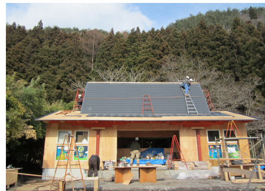
Photo 27: San-San Kitchen House under Construction Note: Photo by author, Mar. 22nd, 2012.
