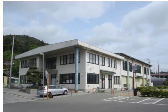
Photo 10: Ofunato District Community Center Note: Photo by author, May 27th, 2013.
