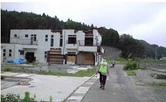
Photo 16 Volunteer work in tsunami devastated area Note: Taken by author
