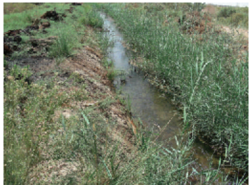
(16) Earthen irrigation canal
