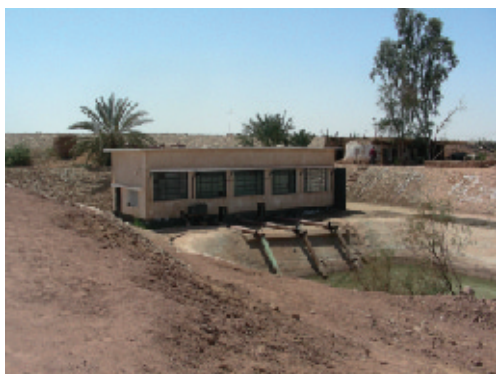
(23) Drainage pumping station (near Rashda)
