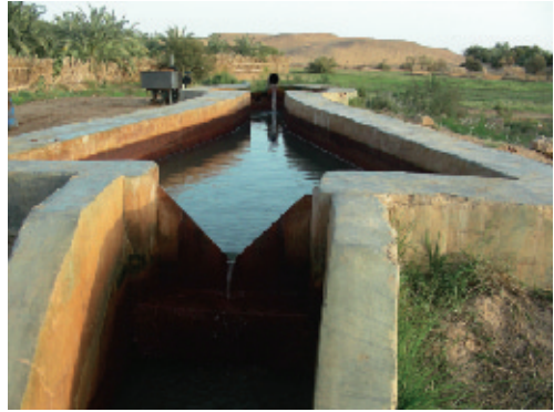
(2) V-notch weir to measure the amount
