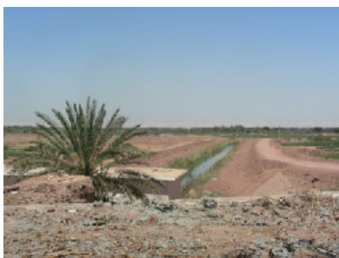
(22) Main drainage canal to a drainage pumping station
