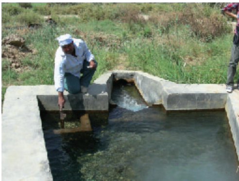
(15) V-notch weir to measure the amount of water
