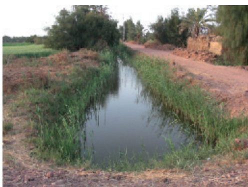
(21) Main drainage canal
