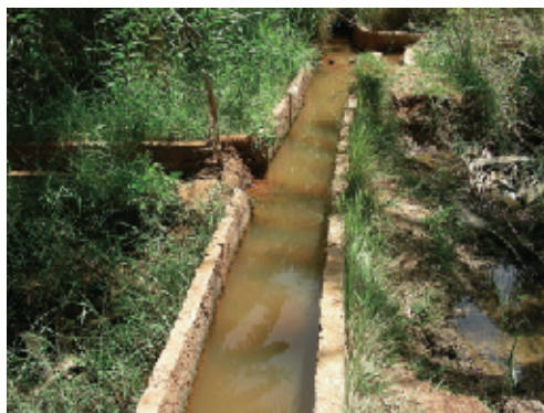
(8) Concrete irrigation canal
