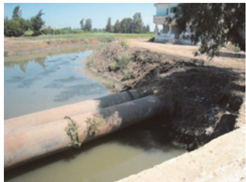
Photo 2-5 Drainage Canal in Sidi Oqba Village (August 2010)
